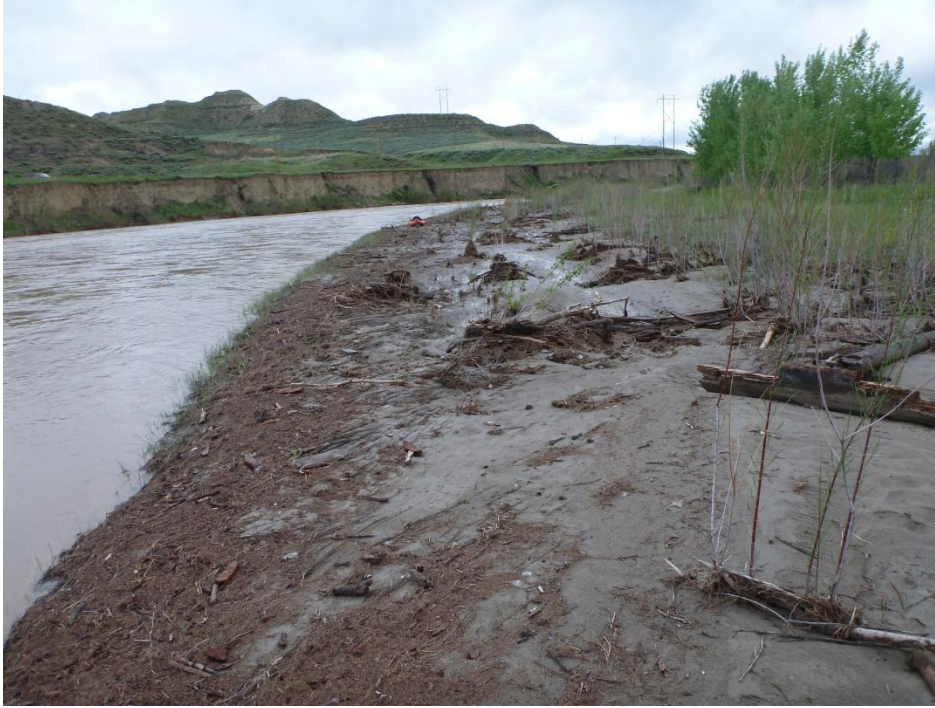
Powder River Site 12 – East Bank. Picture taken facing north.
